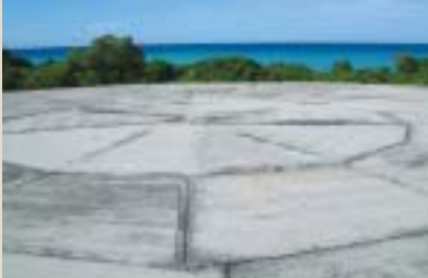
The concrete dome on Runit Island (part of Enewetak Atoll), covering radioactive deposits (photo by Seiichiro Takemine)
