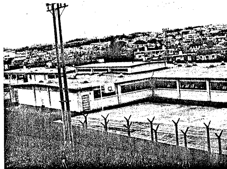
BLDG: 5128 BRIG- TO BE DEMOLISHED
