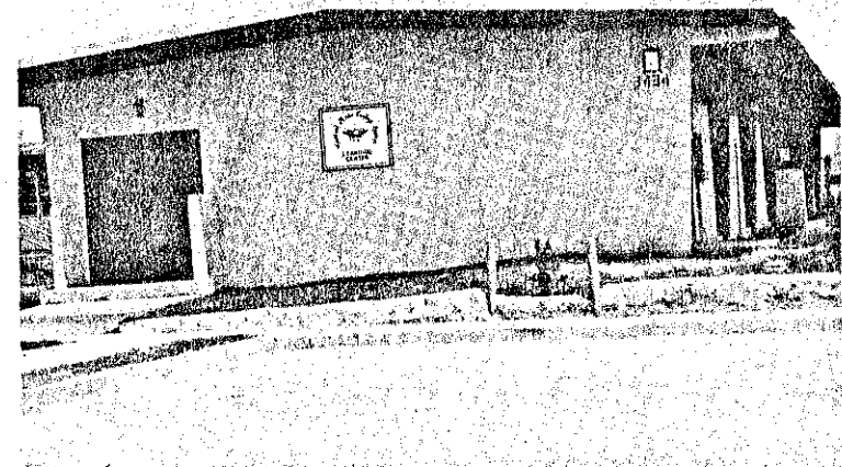
Building 3434, Education Center
