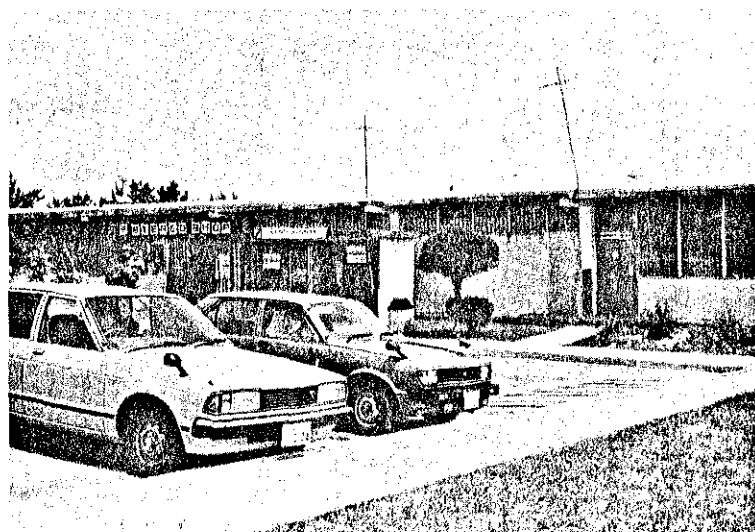
Building 3419, Exchange Outlets
