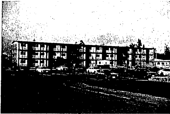
BLDG. 1498, BEQ - BEQ AREA
