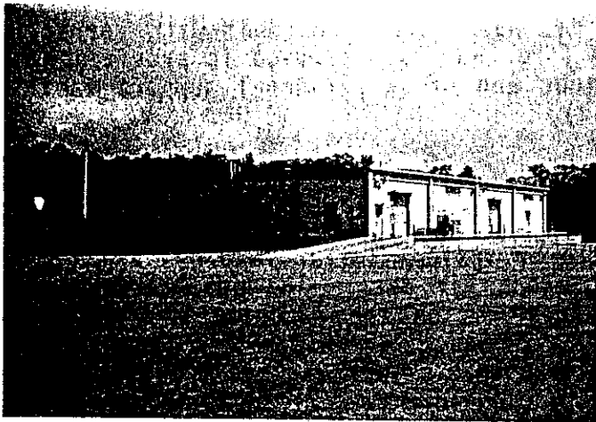
BLDG. 44105, INERT STOREHOUSE - AREA 7
