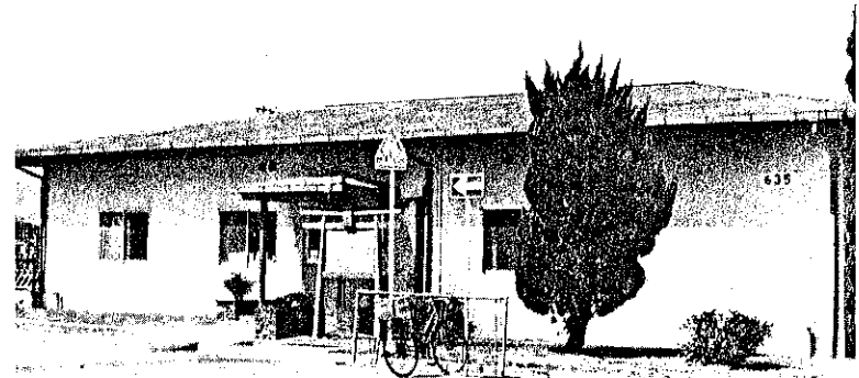
CHILD CARE CENTER BLDG 635
