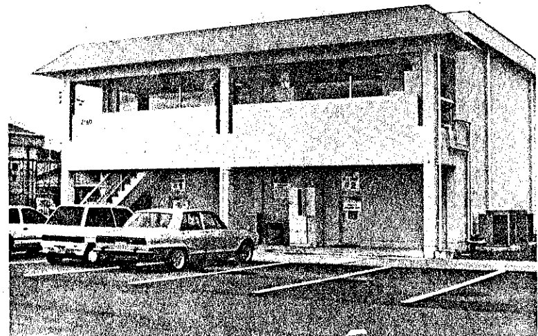
RACQUETBALL COURT BLDG 2160
