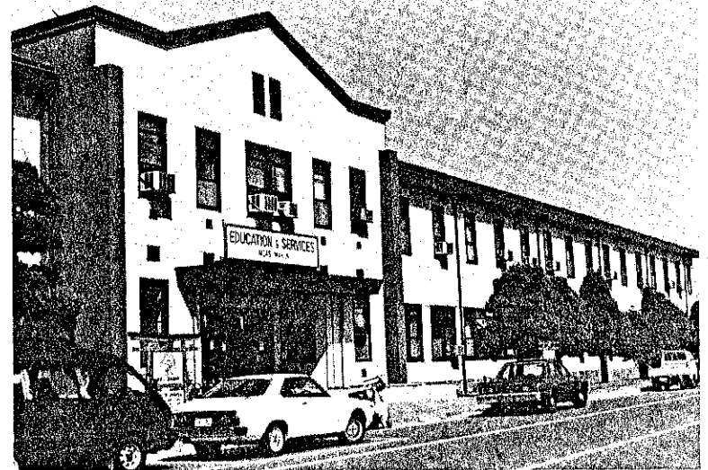
EDUCATION SERVICES BUILDING BLDG 210
