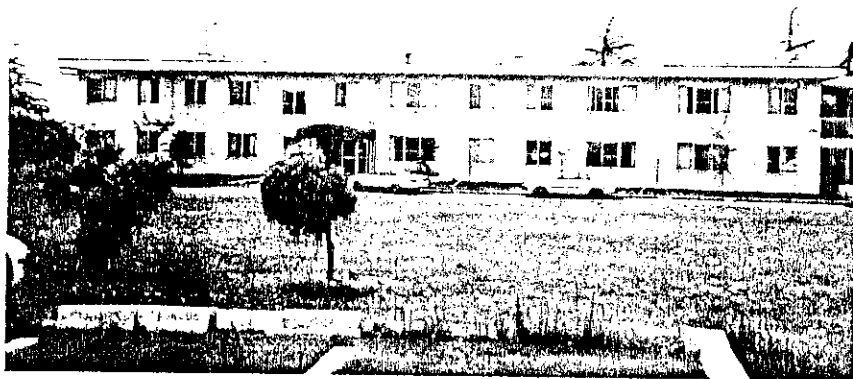
BACHELOR OFFICERS QUARTERS (BLDG 220)
