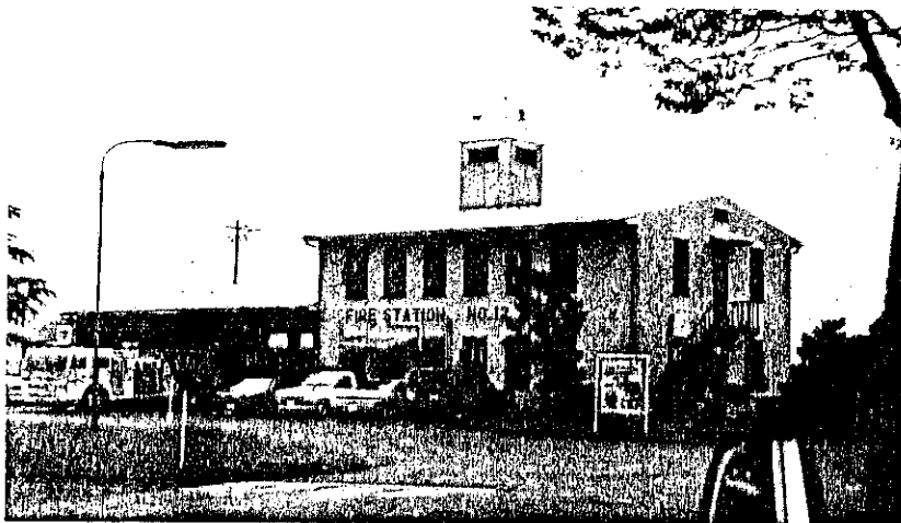
FIRE STATION (BLDG 14)
