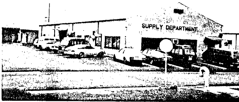
SUPPLY WAREHOUSE (BLDG 16B)
