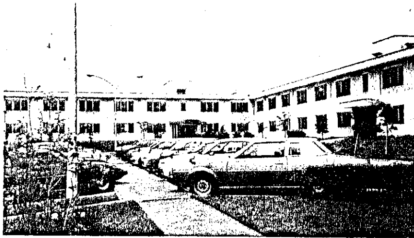
BACHELOR ENLISTED QUARTERS (BLDG 221)
