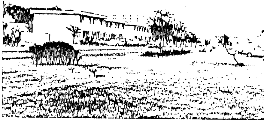
Landscaping to Improve family housing areas
